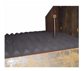
11. Install the nuts and lock nuts, but do not tighten.
