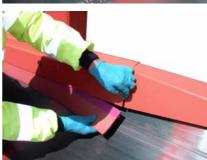
3. Refit clamp fixing screws.
